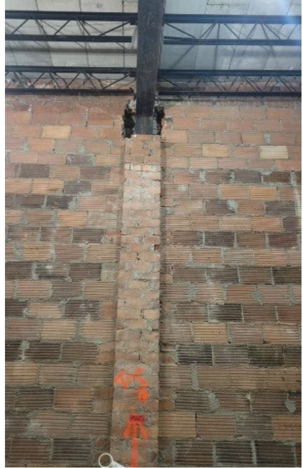
Figure 2 – Interior Wall Demolition
