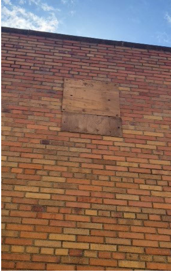
Figure 1 – Exterior Wall Demolition
